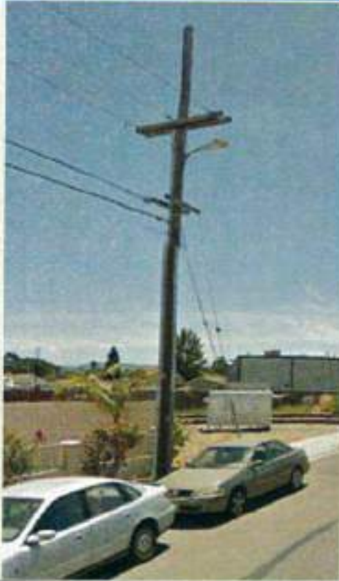
Alternate Pole NORTH #1- Proposed design does not meet GO95 standards for utility poles
