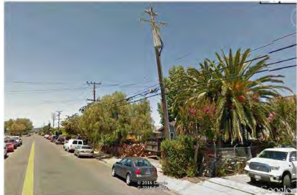
Site will not support design and be GO 95 compliant
