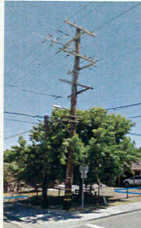
Alternate Pole South #2- Pole will not support proposed design, due to G095 regulations
