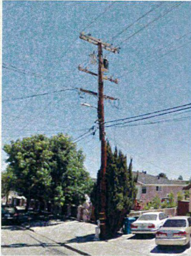
Alternate Pole NORTH #1- Pole will not support proposed design, due to G095 regulations
