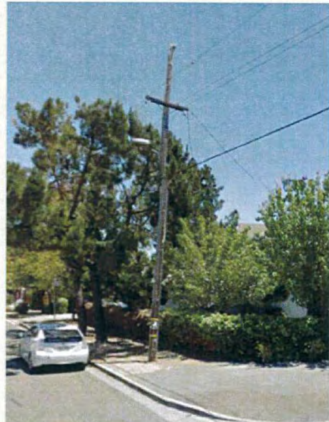
Alternate Pole East #2- Pole will not support proposed design and stay in GO 95 compliance
